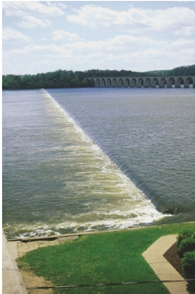
Low head dams, like the one shown above, pose a serious danger to boaters, particularly to paddlesport enthusiasts. These dams are virtually invisible from upstream, plus the hydraulic jump resulting from the water falling over the dam creates a powerful undertow that can trap and hold boats, people and other objects.
